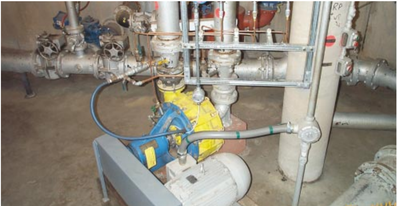
Photo 1. Condition-monitoring peripherals, installed subsequent to the optimization
